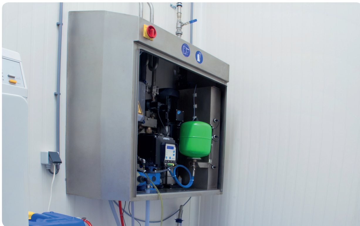
The CFD-Q 64E enables its users to foam and disinfect.
